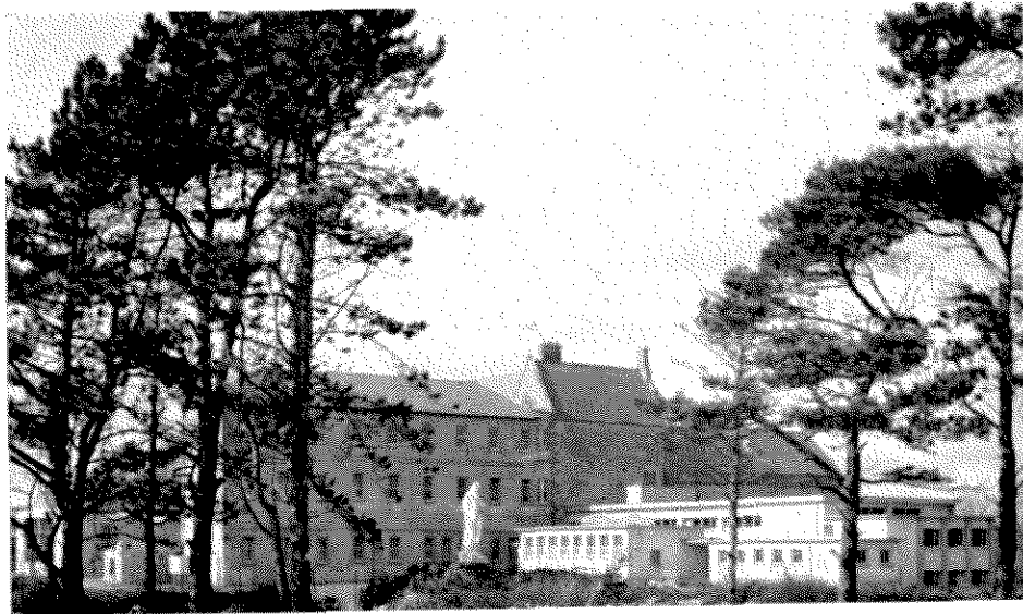
A view of the new East Block
