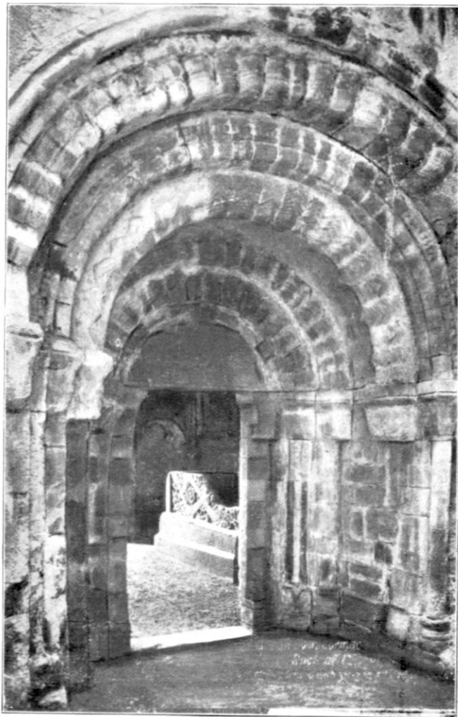
ENTRANCE TO CORMAC'S CHAPEL.
