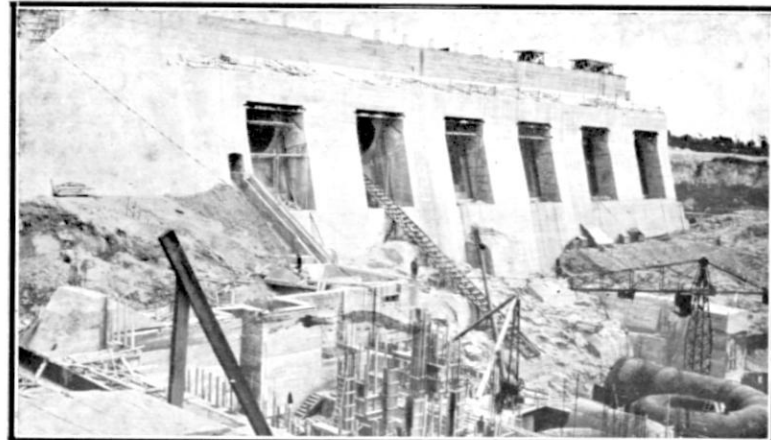
Work on the Power Station.
